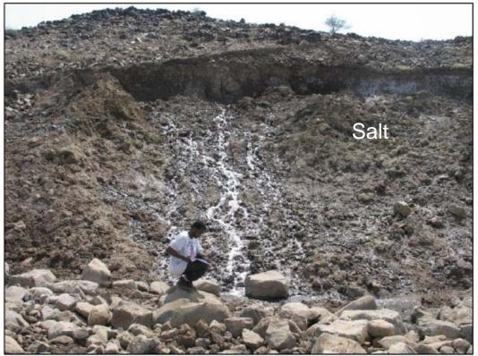
In the US, 20% of Dam failures have been caused by piping (internal erosion caused by seepage)
