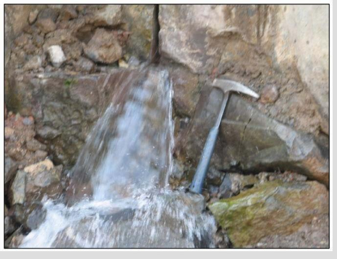
This is leakage through the right abutment after the raining season in 2010. The sever leakage wasn't through the Dam body but the country rock
